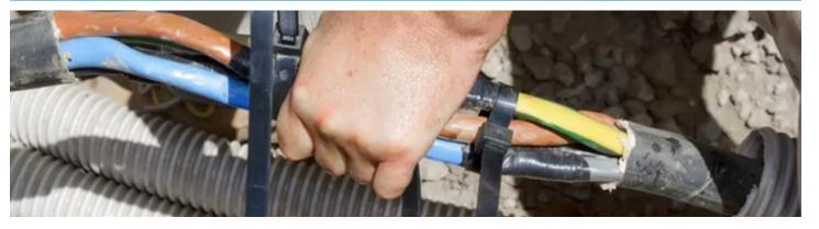
**Cable ties** are simple fastening devices, typically made from plastic. They're not structural and don't provide a pathway for cabling. However, industrial cable ties can still maintain a semblance of neatness in the right setup, especially temporary ones.
